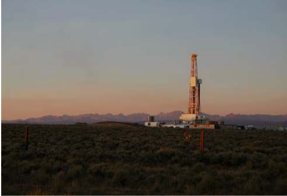
A drill rig near the town of Pinedale, Wyo. (Credit: Abrahm Lustgarten/ProPublica)
